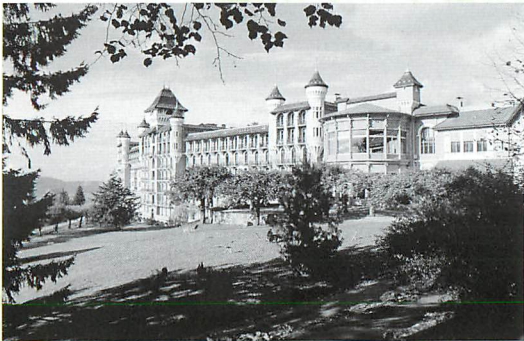
The former Caux-Palace Hotel is now an international conference centre for Initiatives of Change
