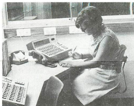
The new telephone switchboard Photo: Azzopardi
