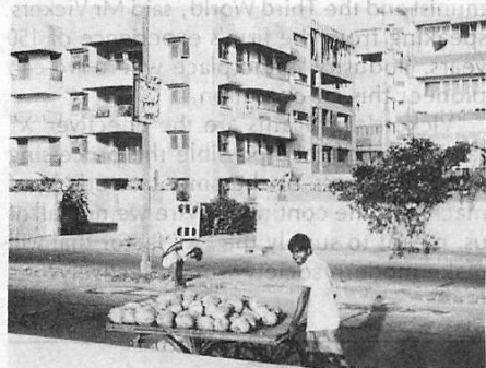
New MRA flat—the unfinished building (centre right).
