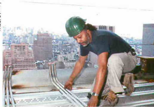
Laying electrical conduit at the top of the World Trade Center
