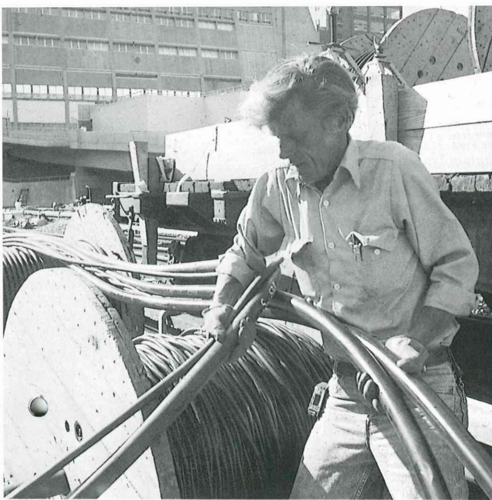
Feeding power cable into a manhole at Long Island railroad yards
