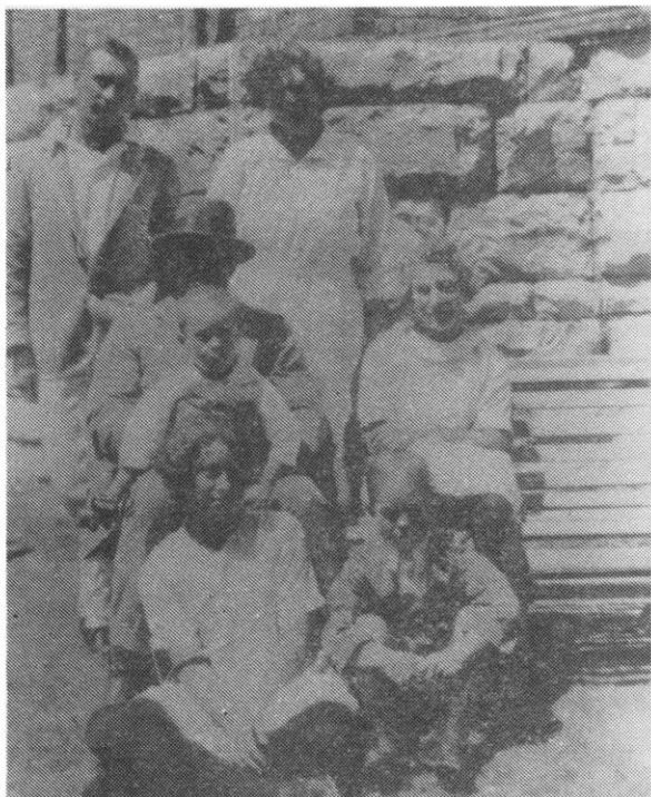
RBK, mother Norah, Pannell with Con, Enid, Joyce, Keith in 1923 on building site.
