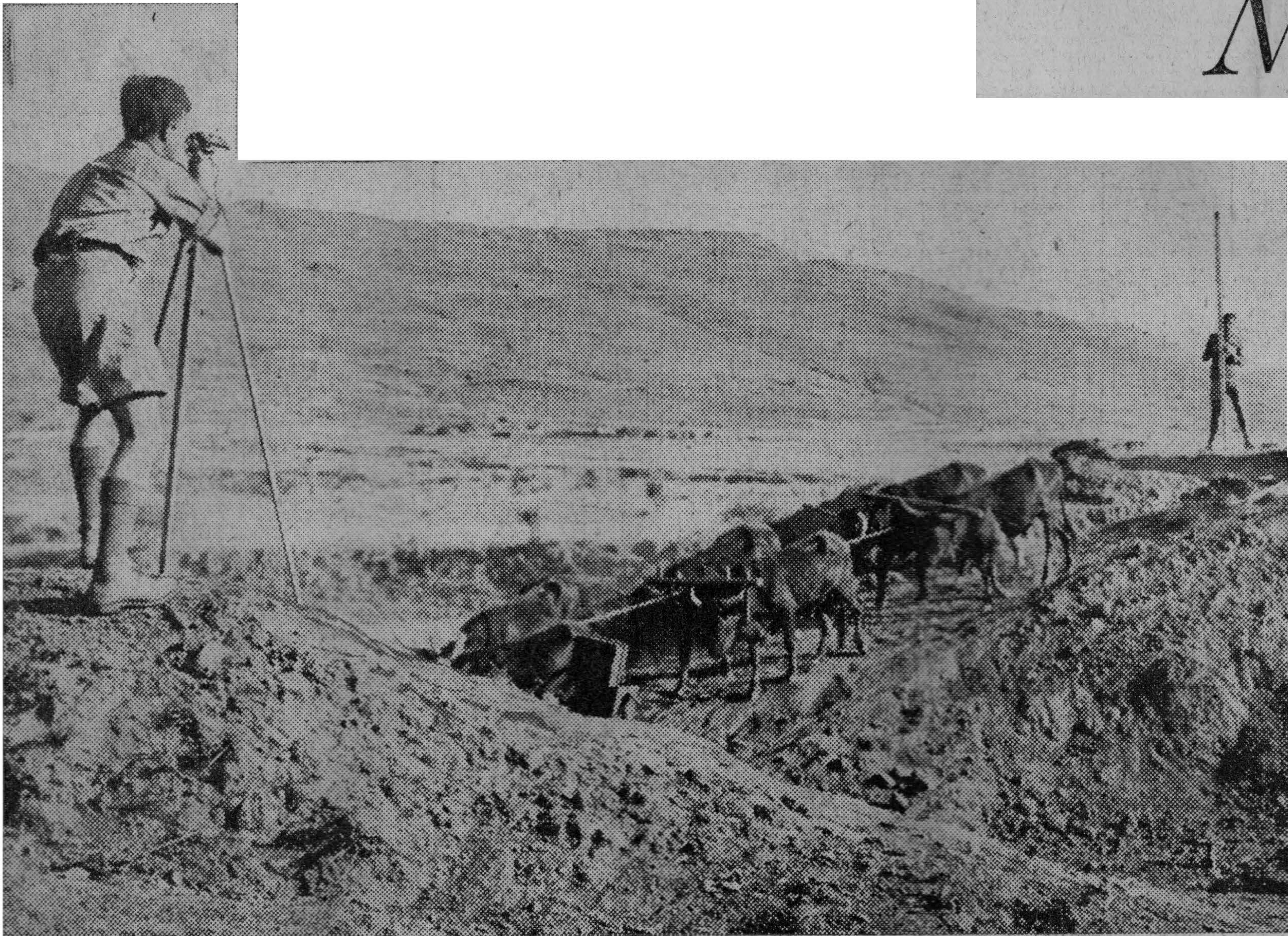
TAKING THE LEVELS on a Rietvlei farm, where 20 young South Africans are building a dam. The oxen are dragging down another load to the growing earth wall.
