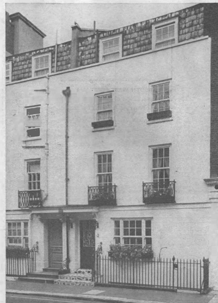
No 3 Culross Street, Mayfair: completely renovated and modernised.
